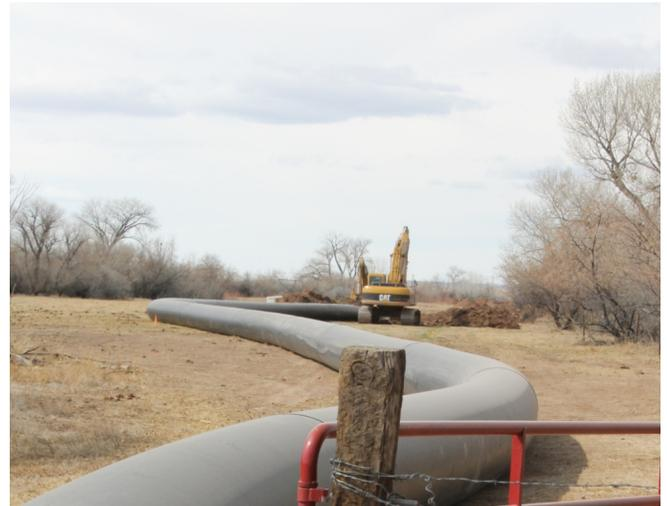
**Sections of large-diameter PE 4710 HDPE pipe were fused together to make a leak-free line that runs 21 miles to provide water under pressure to irrigate some 53,000 acres of farmland in northeast Utah and saves \$50,000 annually. The undertaking was named Project of the Year for the Plastics Pipe Institute's Municipal and Industrial Division.**
